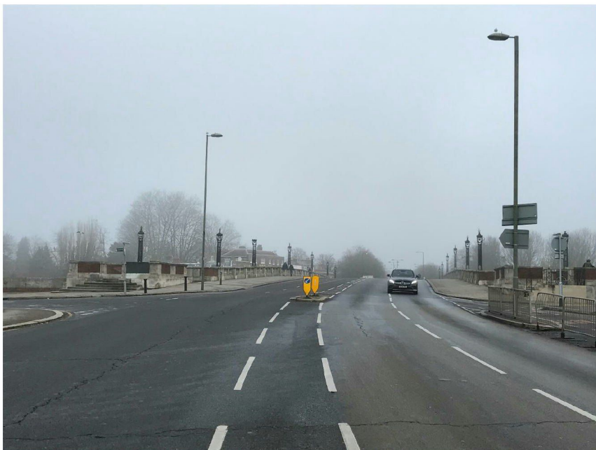
12. View approaching from the south Surrey side. Note the simplicity of the highway layout and the lack of highway or other street furniture within the curtilage of the bridge including on the footways and highway. The 8m street column to the left is the only exception which could be argued is outside the curtilage of the listed structure. The yellow bollards are not sited on the bridge structure but the detriment to the setting of the bridge is dramatic.
